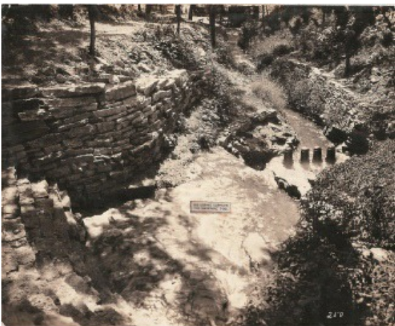
Four hydraulic rams moved the water from the Big Spring through pipelines to the lodges and cabins all over the original Lake Bella Vista resort.
